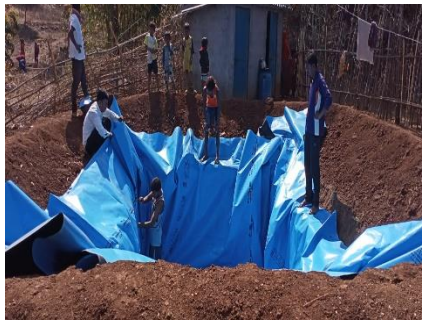
2) Laying out the plastic lining and pitching
